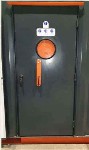
Blast room observation window
